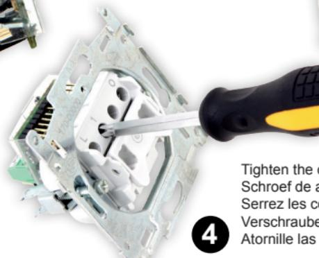
Tighten the connections with a screwdriver.
